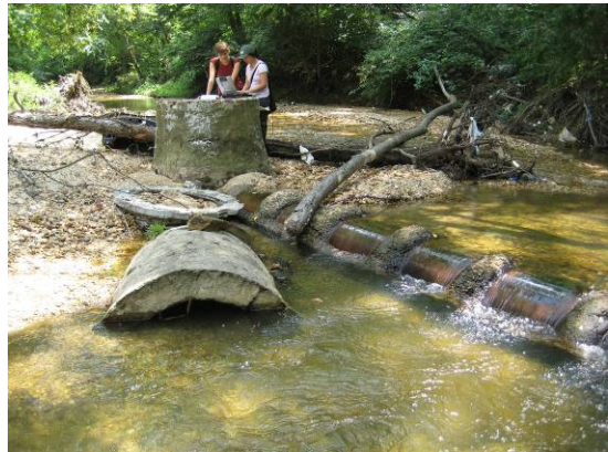
Degraded Sewer System infrastructure in Oxon Run
