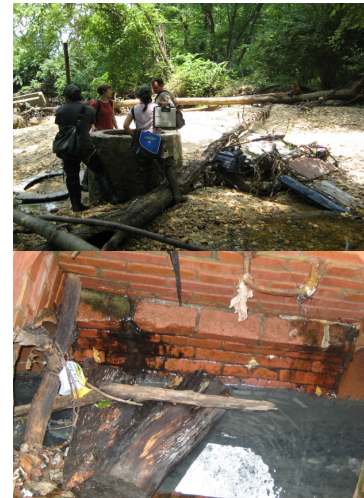
Exposed sewer line infrastructure
