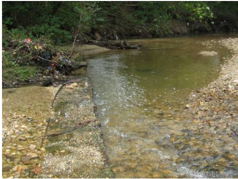
Sewer line crossings can be barriers to fish passage
