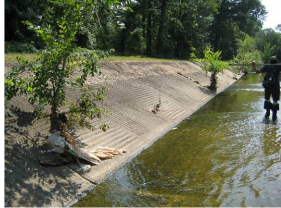
Approximately 1.5 miles of Oxon Run, within the District, is a concrete lined channel
