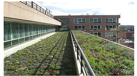
Green roof at the Reeves Center.
